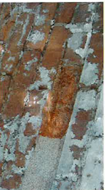
Sandblast or use of high-pressure power washing to clean masonry can scar masonry surfaces, allowing moisture to penetrate.
