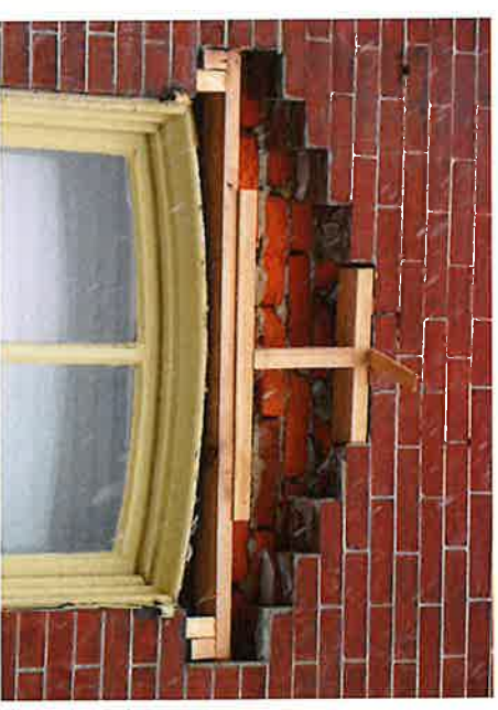
Before: Wood lintel has rotted, causing brick to settle.
