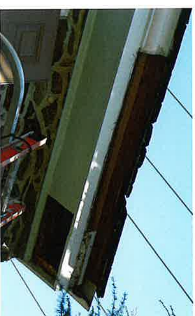
Before: Minshall House cornice repair
