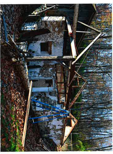
Before: Stucco has come off, exposing the stone to weather conditions.
