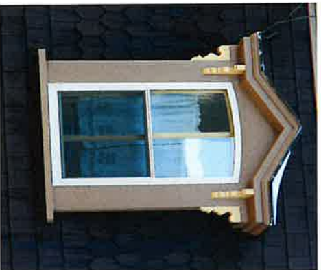
Recommended: This new storm window protects the original window while matching its shape.
