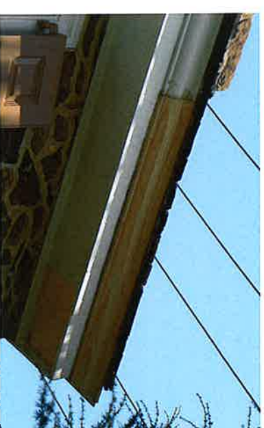
After: Minshall House cornice repair
