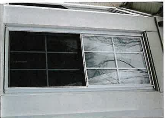
Not Recommended: Vinyl replacement window with inserted grid lacks articulation of a true divided-lite window or appropriate trim.
