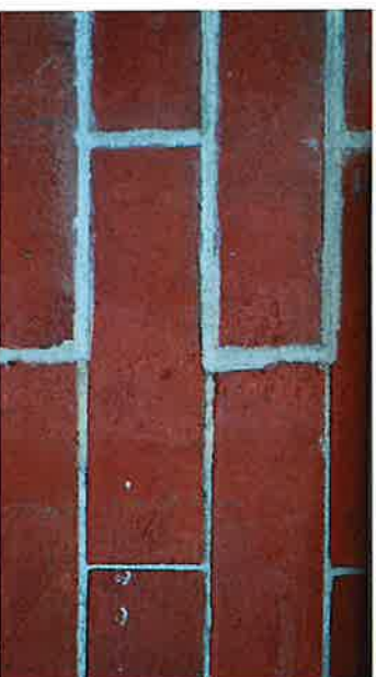
An example of improper joint width, color, and joint profile on left.
