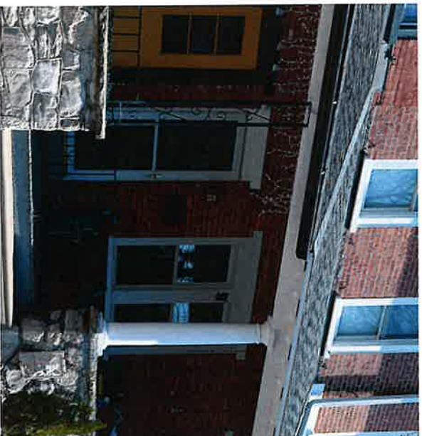
Not recommended: Original wood posts should not be replaced by decorative metal.
