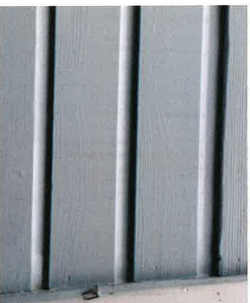
View of repaired and repainted wood siding.
