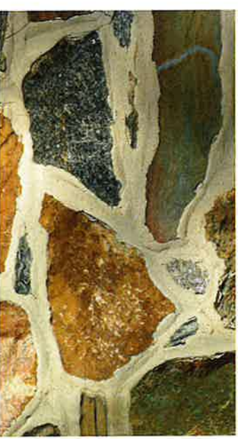
An example of appropriate repointing in this stone wall.
