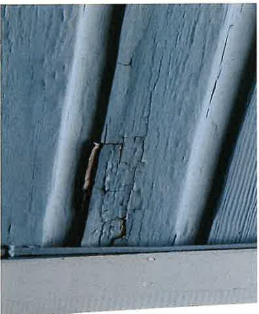
Regular painting protects wood surfaces. Paint failure has led to rotting wood siding.
