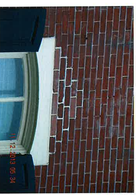
After: New wood lintel and brick reinstalled.
