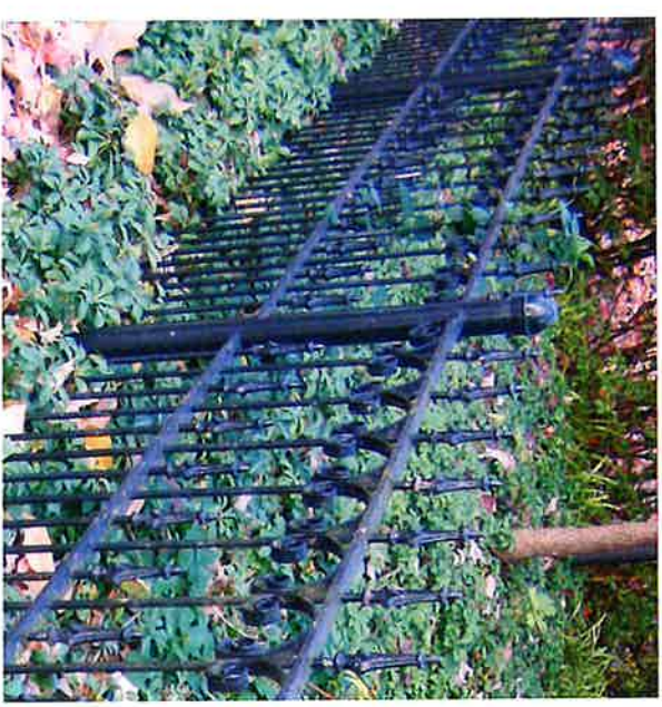
Recommended: Original fence posts have been replaced to support original wrought iron fence.
