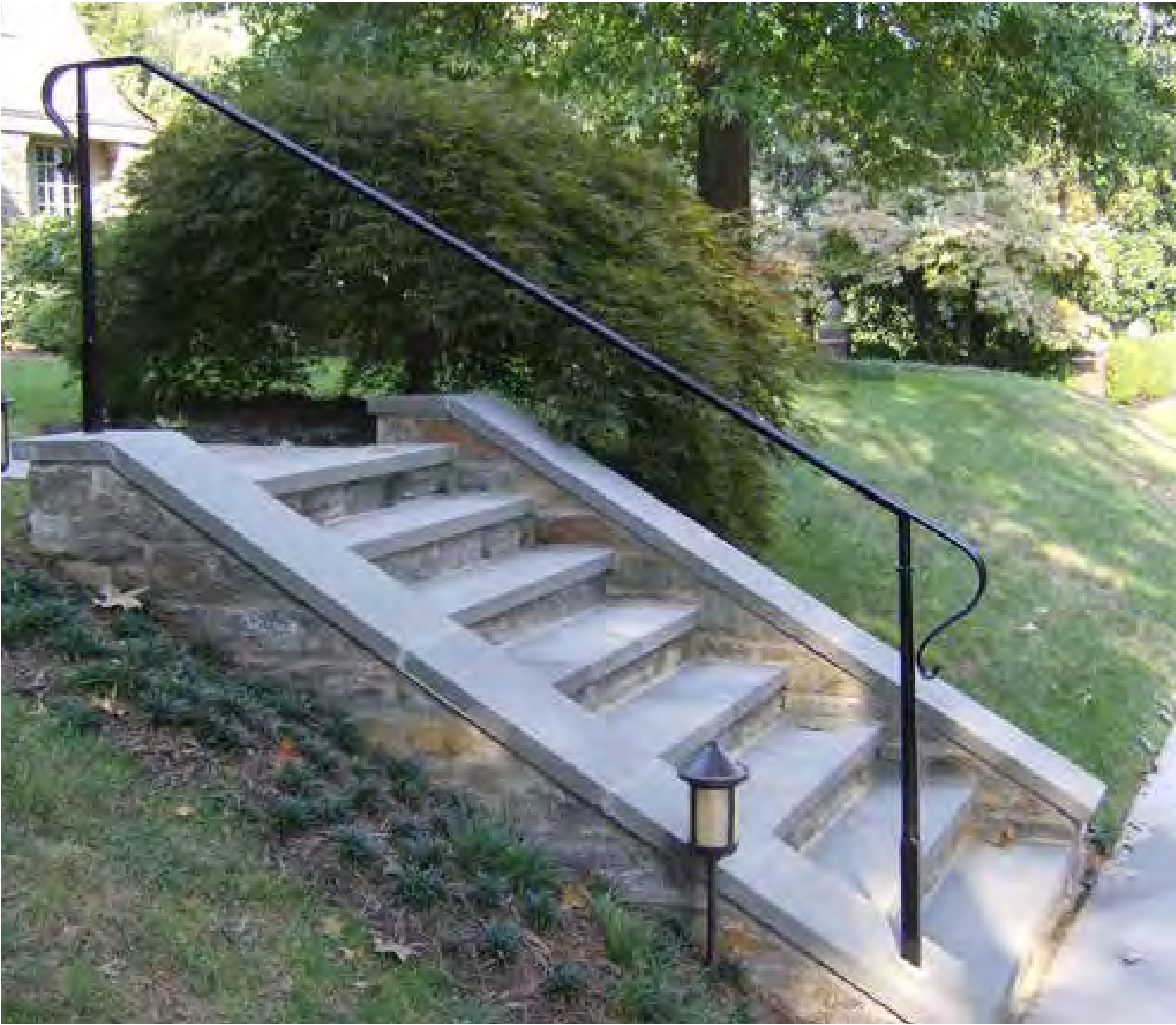
Steel Handrails, Powdercoated Black
