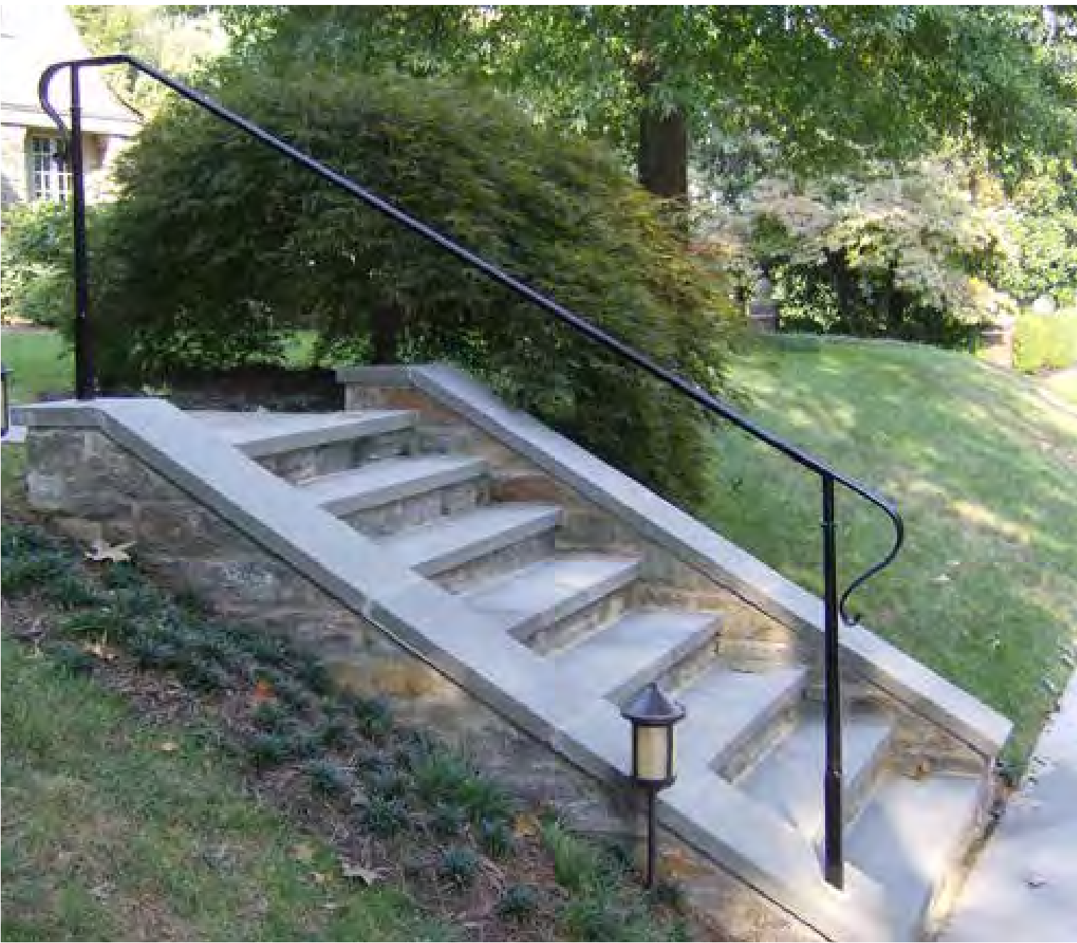
Steel Handrails, Powdercoated Black
