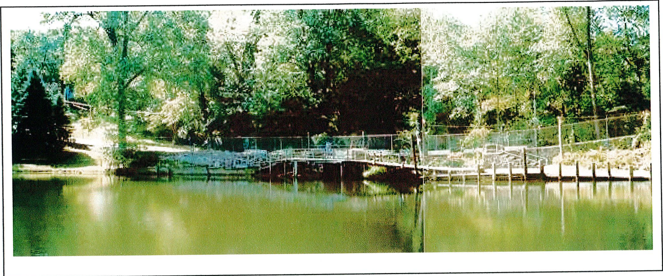
Broomalls Lake and upstream side of bridge/dam. View is looking south.
