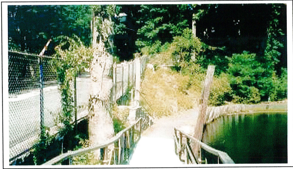
Upstream walkway along edge of lake and above culvert level.
