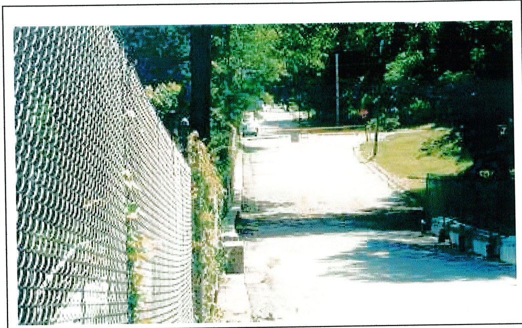
Roadway looking east.
