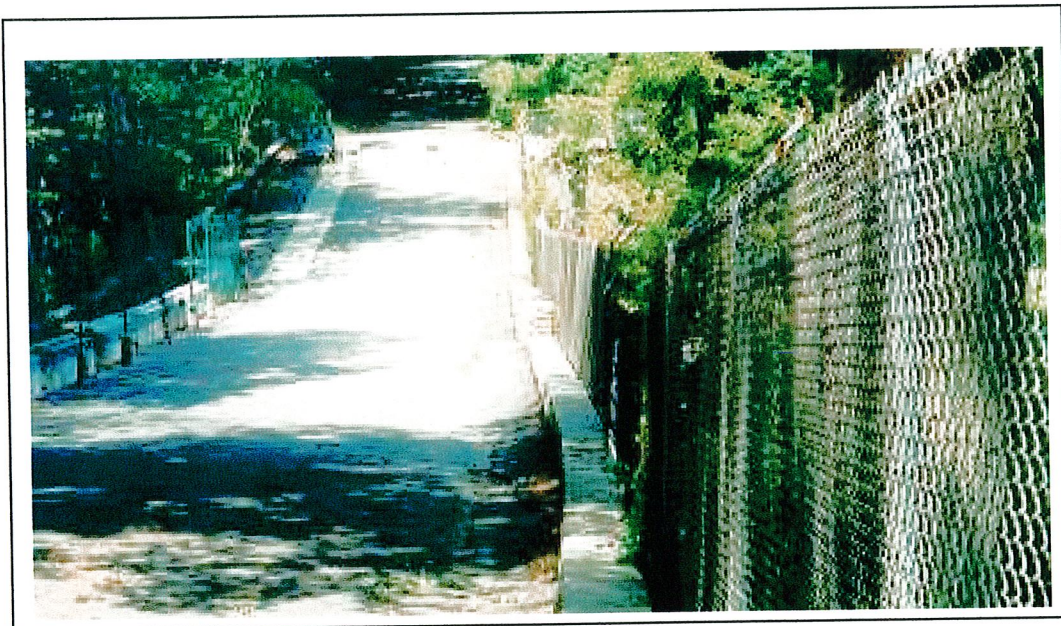
Roadway looking west.
